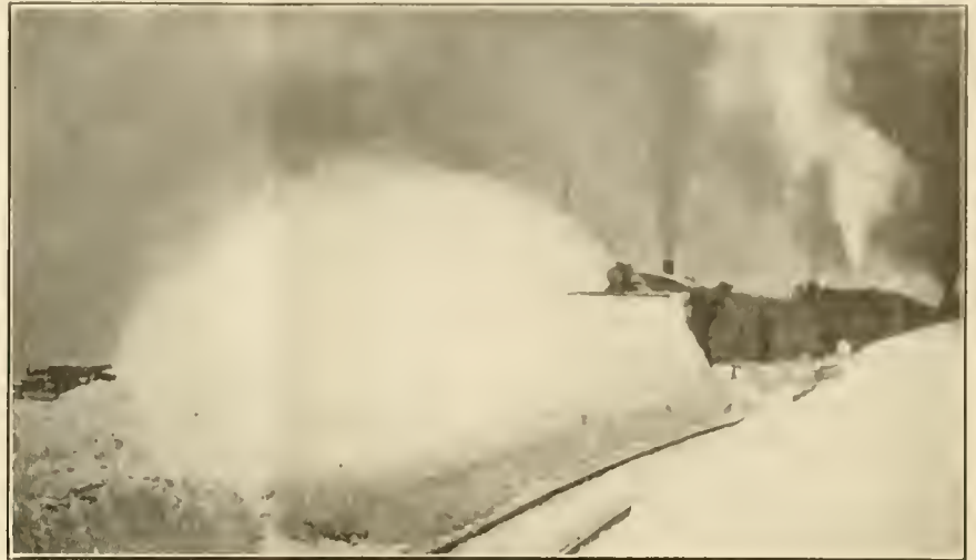
ROTARY SNOW PLOW CLEARING A SIDING.
